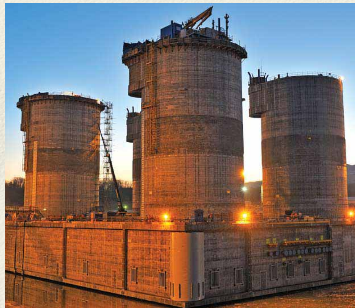
GBS is ready to move from Nakhodka to the North of Sakhalin
