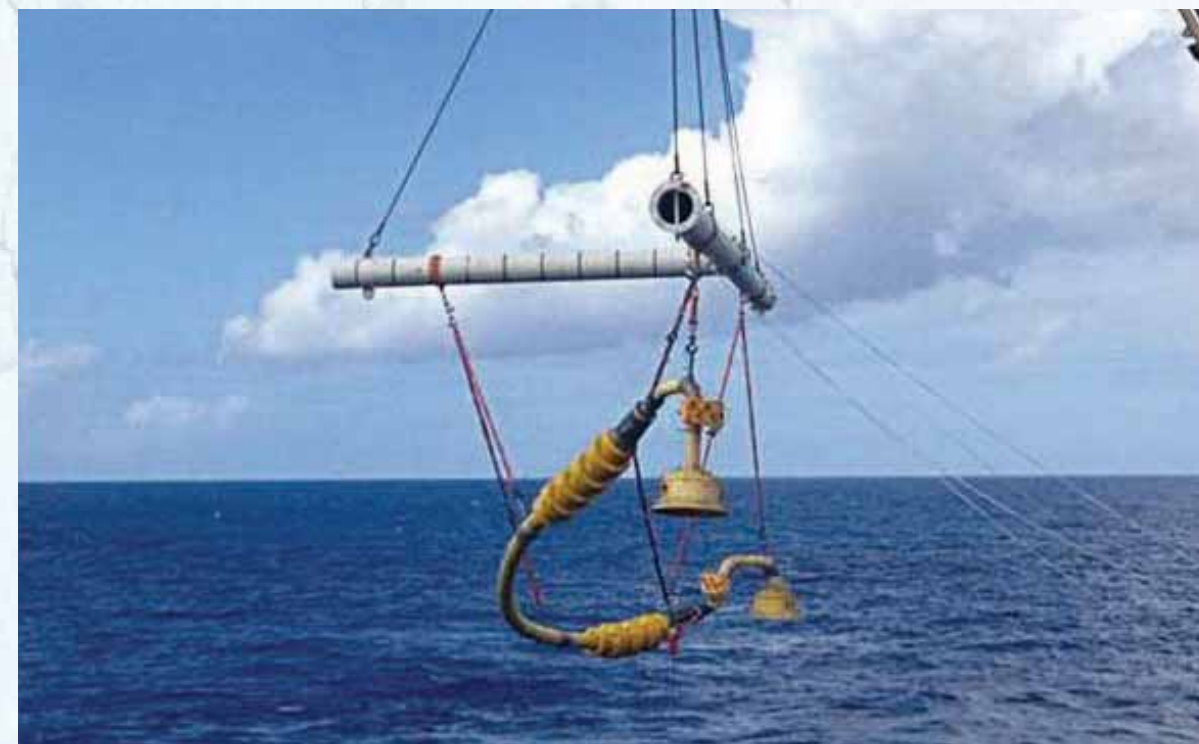
The flowline production jumpers being deployed, Brazil
