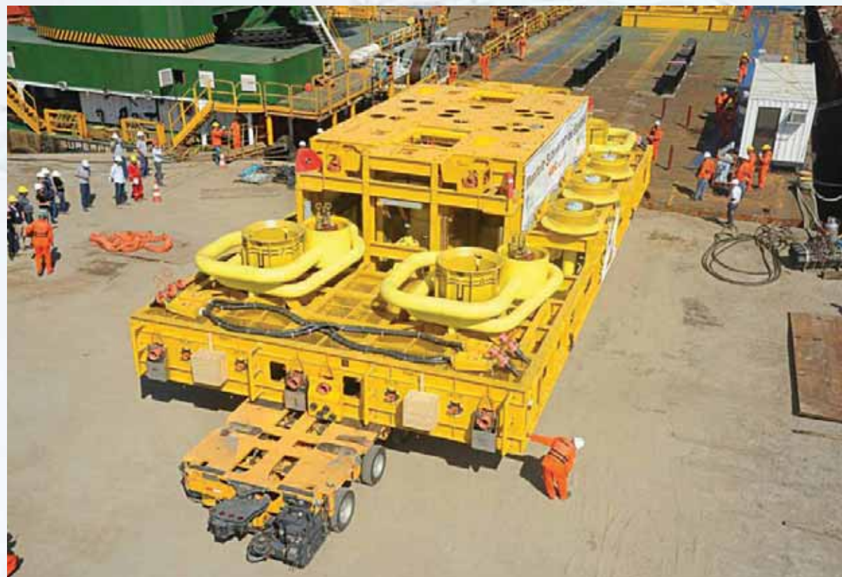
ALM #3 being loaded to the barge – prior to their load out to installation vessel, Brazil
