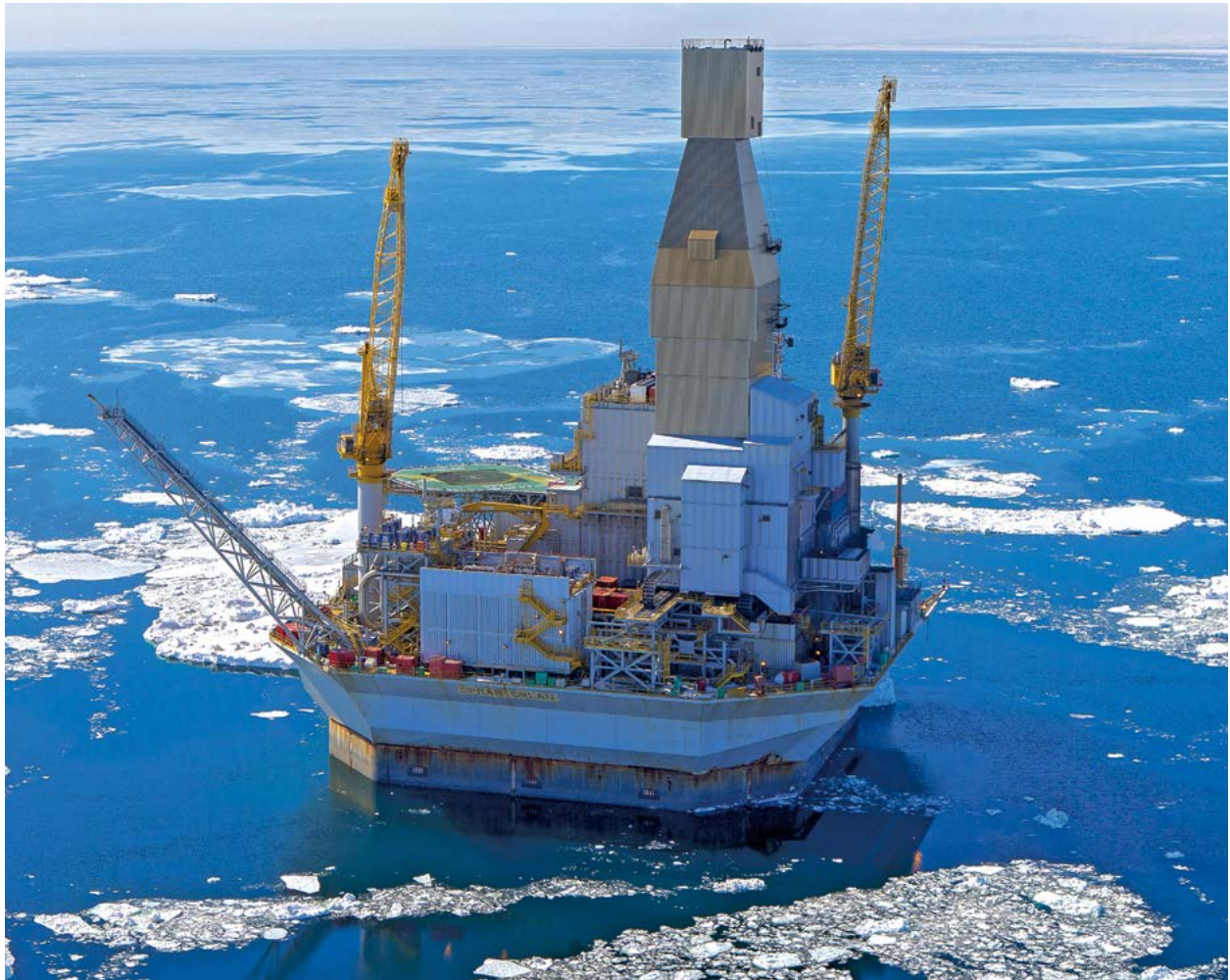
Orlan Platform, Chayvo Field, offshore Sakhalin Island, Russia a Ice-resistant offshore platform capable of drilling Extended Reach Drilling (ERD) wells
